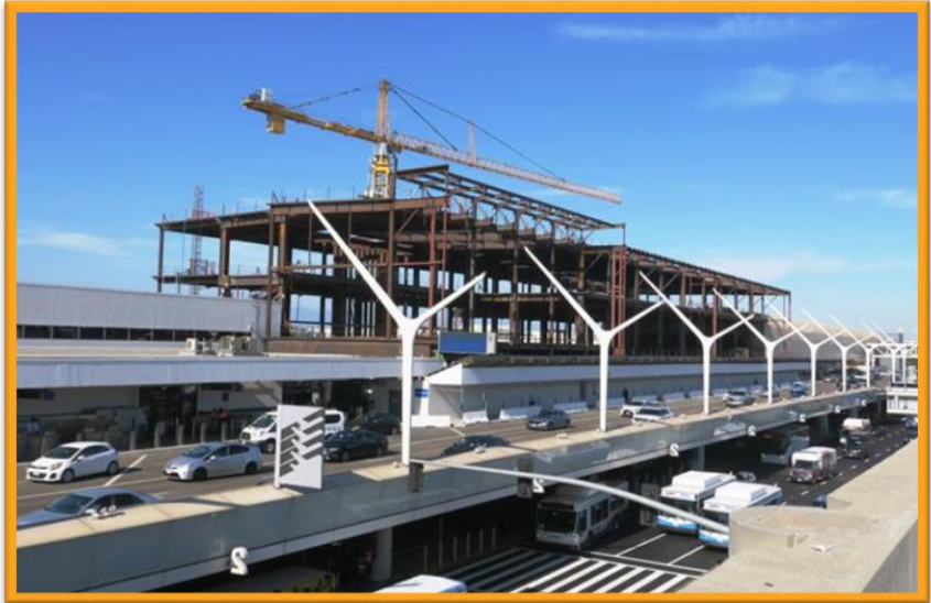
Terminal 1.5 Structural Steel
